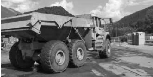
Hauling material across Railroad Avenue in late July.
