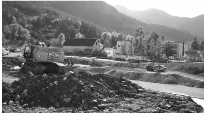
Excavation and backfilling on 5th Street and surrounding areas in mid-September.
