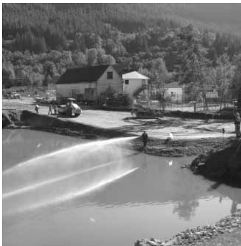
Crews use hoses to push oil into areas where it can be collected and recovered.
