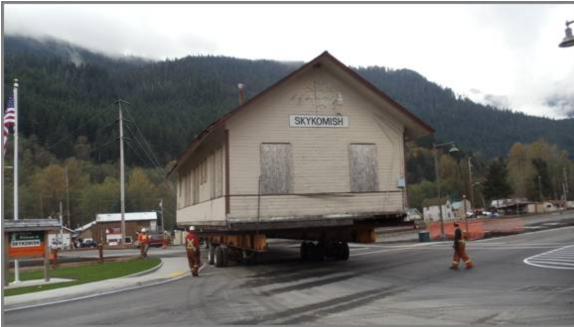
Photo: The Depot Building is moved down Railroad Avenue and across the 5 th Street crossing to its new location on the rail yard [11/04/11].
