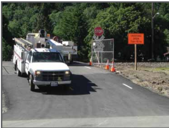
Construction of a temporary railroad crossing
