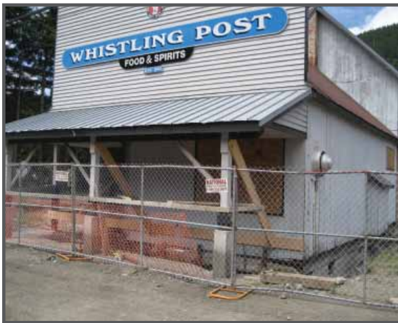
Whistling Post preparation for relocation
