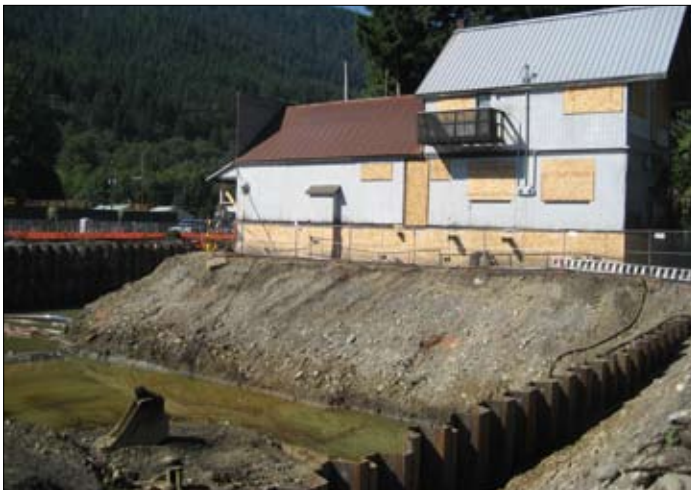
Excavation under the Whistling Post's original location.
