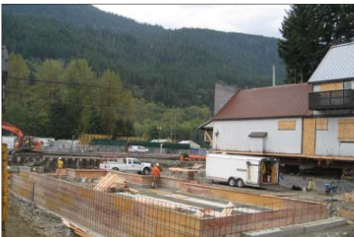
Crews construct the footings and foundation for the Whistling Post.
