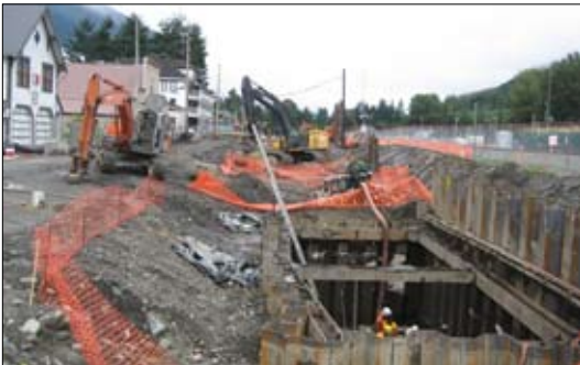
Crews use sheet pile to prepare for HCC vault installation.
