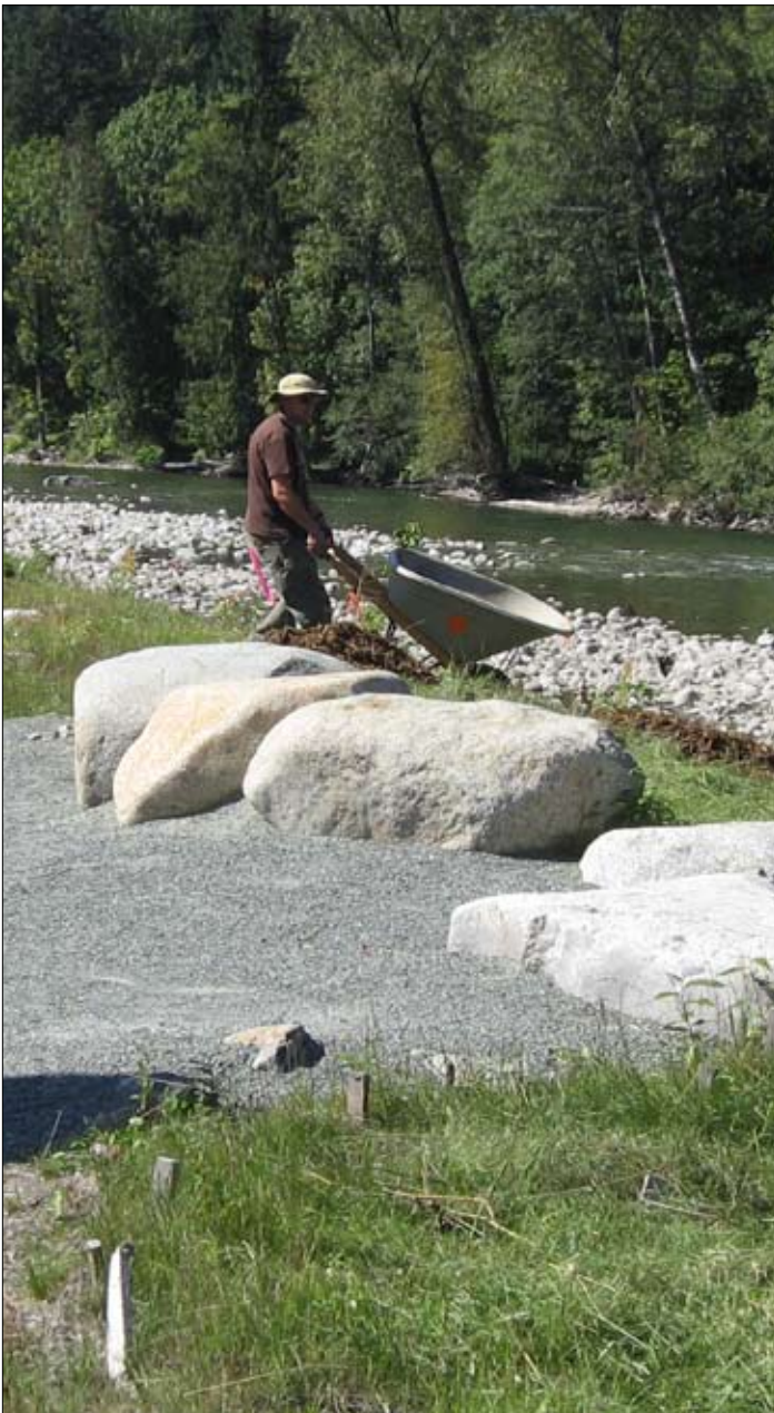
Crews work on levee restoration and plant maintenance.
