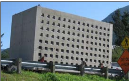
The first concrete vault for the HCC system arrives in Skykomish.
