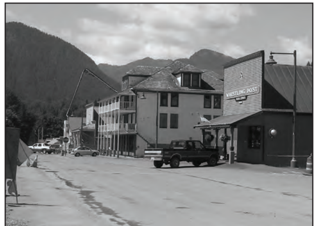
Looking west along Railroad Avenue during restoration activities in August.
