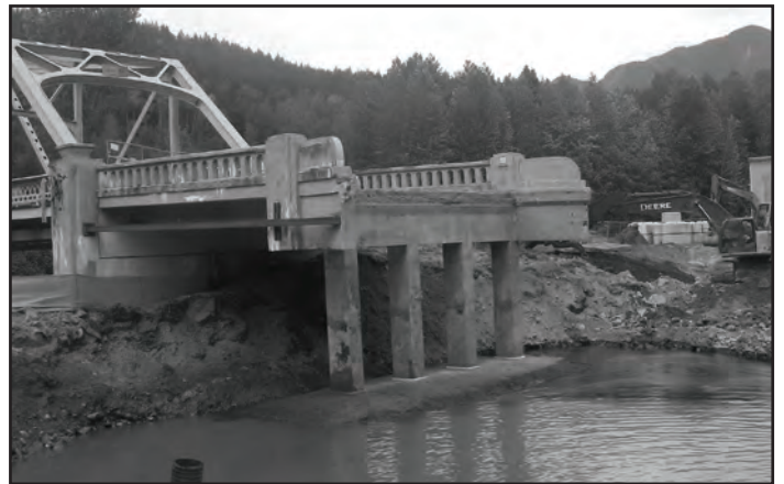
View of bridge abutment during 5th Street Bridge closure and excavation.
