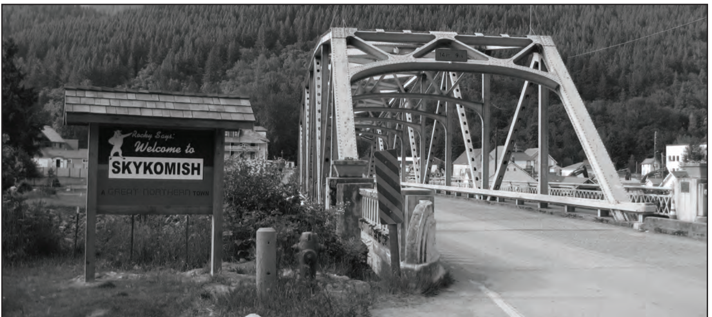
5th Street Bridge open to traffic.
