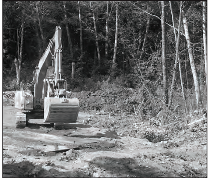
Clearing and grubbing prior to FMC West Wetland excavation.
