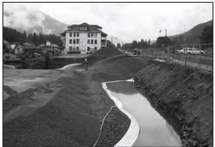
Excavation and oil recovery in the NWDZ.
