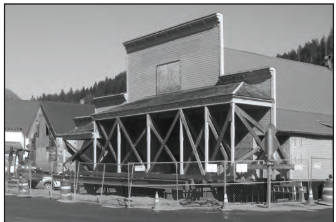
Bracing on Maloney's General Store helped protect the building during relocation.
