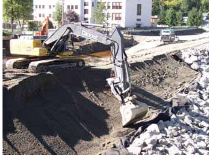
Rebuilding the levee.
