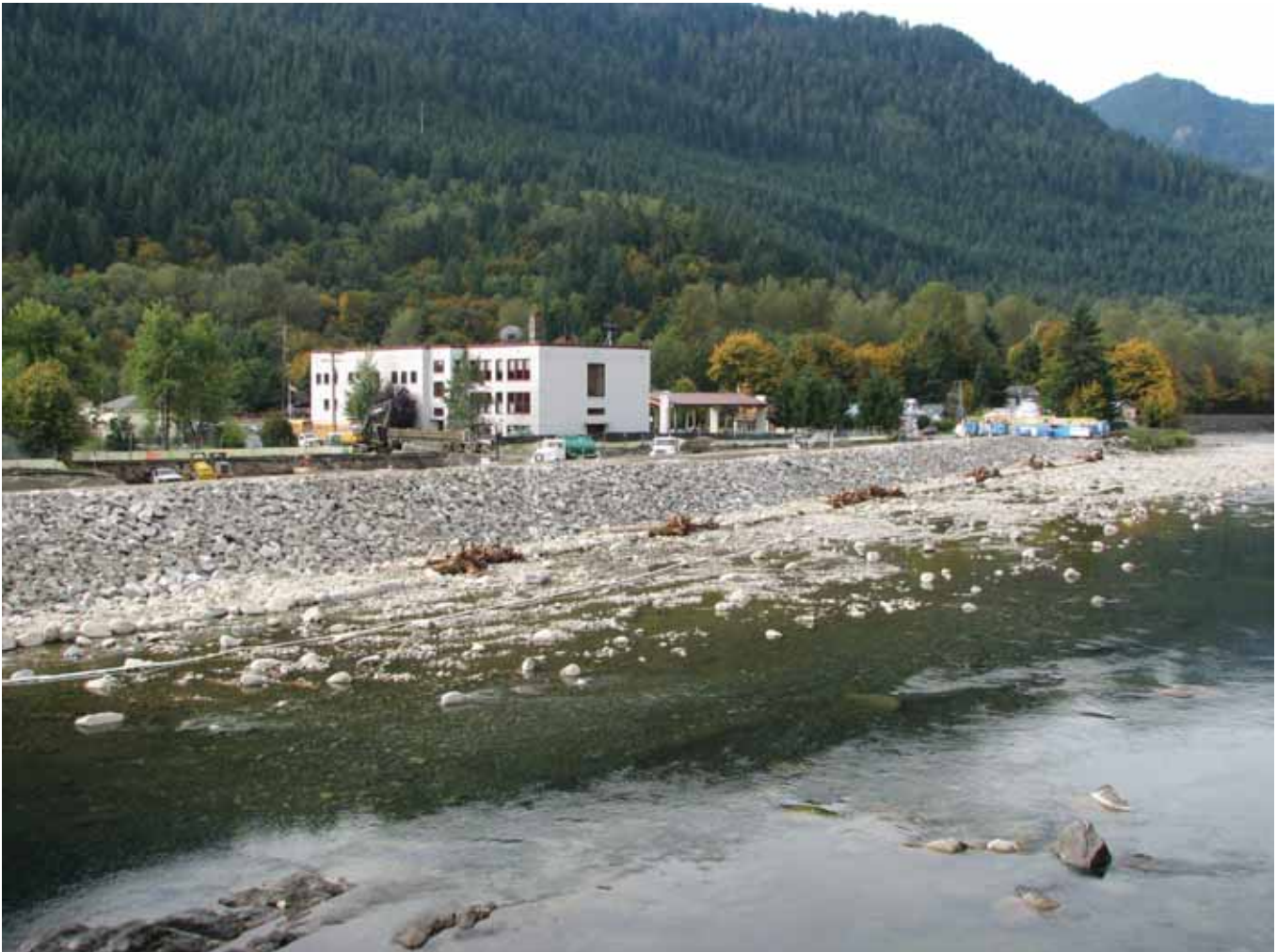
Levee progress as of October 3.
