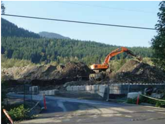
Stockpiled excavated material.
