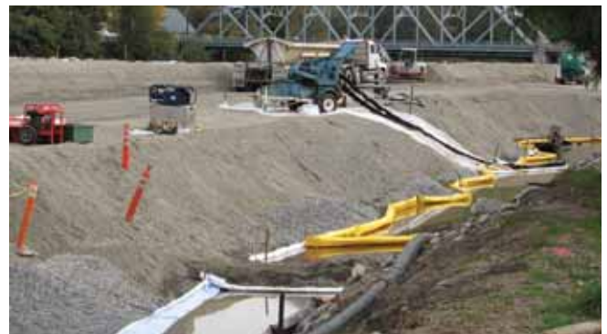
Oil recovery in the shoring wall trench.
