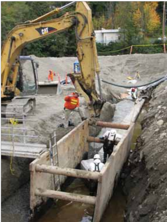
Shoring wall construction.
