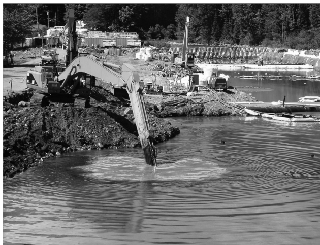
Excavation highlights the oil layer contained inside the cofferdam
