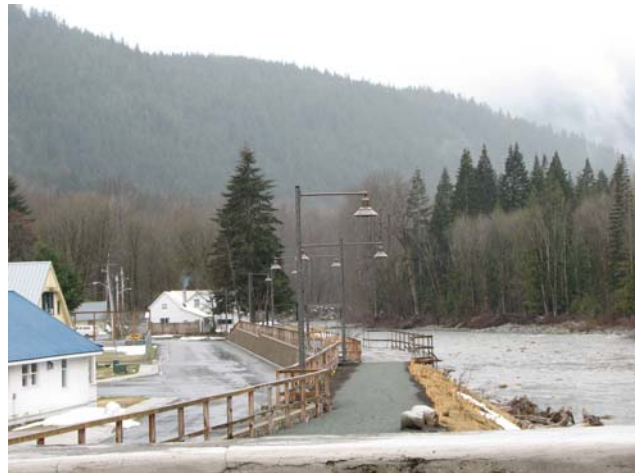
New levee lighting
