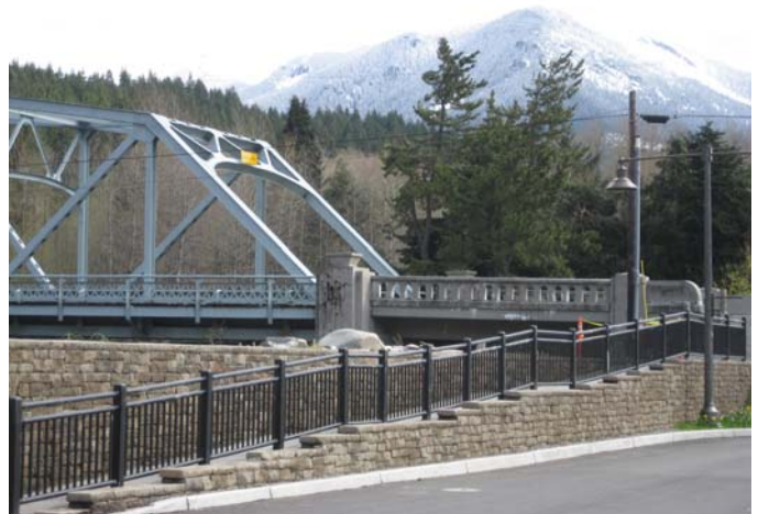
New levee railing
