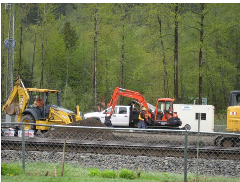
Rail yard excavation
