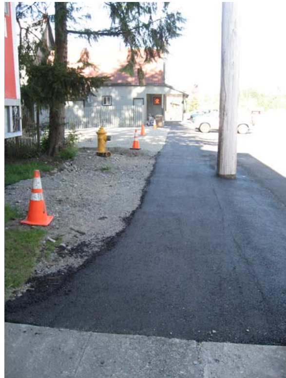
Temporary sidewalk and booth area installed for the Centennial.
