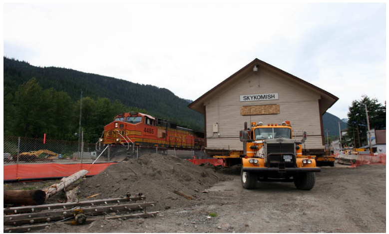
Moving the Depot
