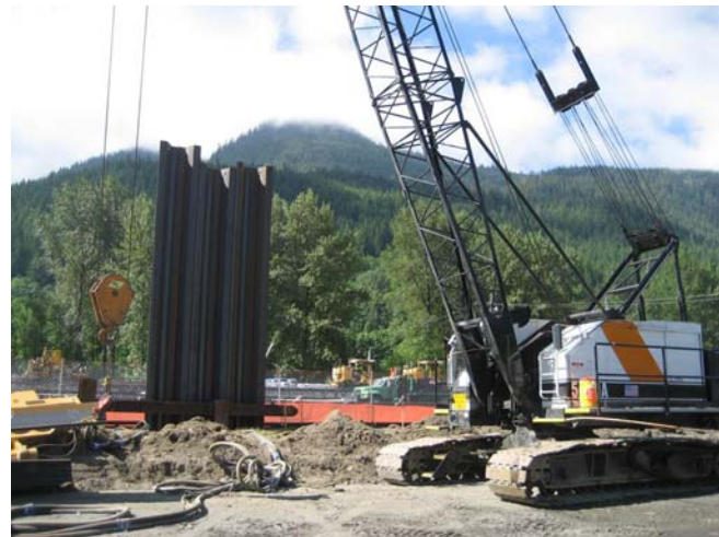
Sheet pile installation.
