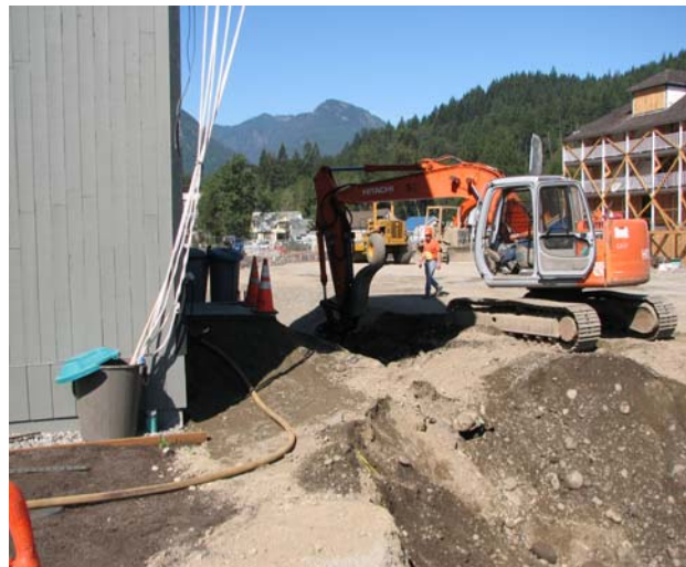
Preparing for sheet pile removal behind the Whistling Post.
