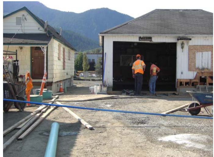
Restoration work last week at the Sarno and Martin houses
