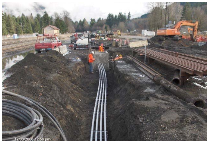
Crews install piping for the HCC system.
